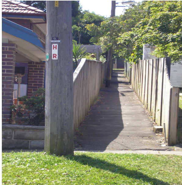
Image 35- View of drainage reserve from Howell Place to Matthews Street looking north (127/10084)
