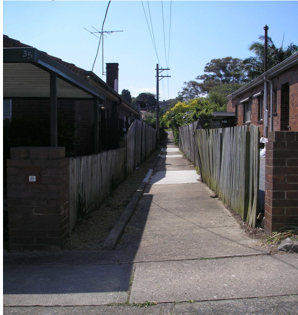
Image 34- View of drainage reserve from Bridge Street to Howell Place looking north (128/10084).
